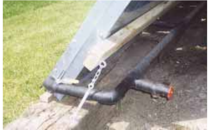
The three Yazaki panels are anchored to railroad ties.
