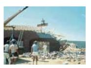
Placing too big a pile of sheathing on an unbraced truss roof can lead to disaster. Amazingly in this case, the falling dominos were halted when a quick-thinking carpenter was able to brace the remaining upright trusses before the collapse reached the part of the roof where he was working.
