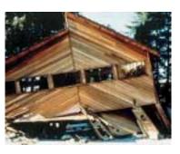
Because the tiny return walls on each end of the three-car garage could offer little resistance, lateral loads from an earthquake literally twisted this house off its foundation. The structural integrity of the rest of the house was largely unaffected.
