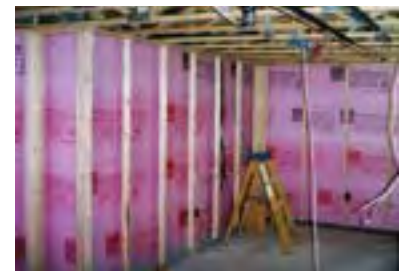
Photograph 8 Unfaced extruded polystyrene against basement wall
