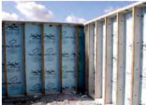
Photograph 11 Pre-cast basement walls with XPS foam insulation
