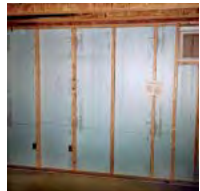
Photograph 9 Unfaced extruded polystyrene against basement wall
