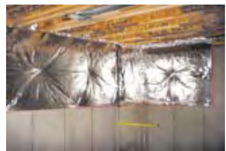
Photograph 4 Blanket insulation with impermeable aluminum foil interior surface
