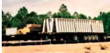
Photograph 10 Pre-cast basement walls
