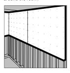
Apply lower row of panels so that tapered edges meet with those of top row. Vertical joints should be staggered. Avoid vertical joints directly above or below a window, door or other opening for best decorating results.
