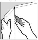
After cutting the panel, smooth the cut edge with sandpaper wrapped around a block of wood such as a piece of 2x4 lumber. Be sure to keep edge as square as possible. Always wear a dust mask when sanding.
