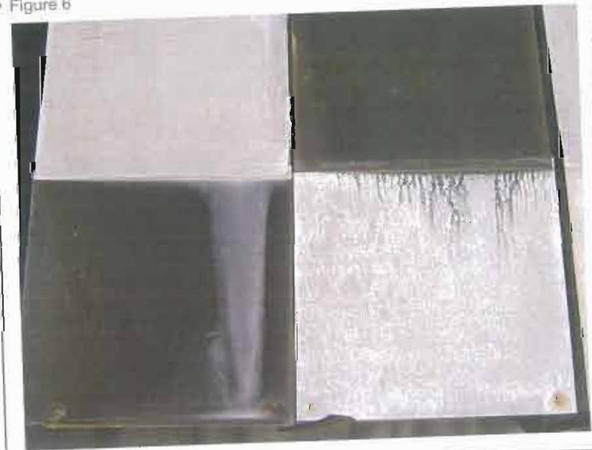
Heavy black streaking occurred on the lead-coated copper sheet below the copper.
