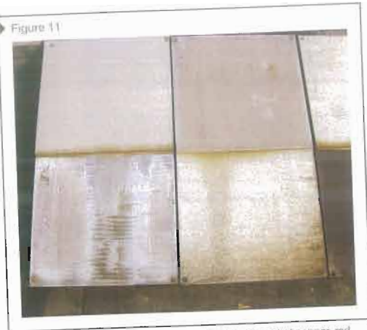
Figure 11 When pairing aluminum/zinc-coated steel with lead-coated copper, red rust occurred at the lock of both sample orientations, indicating failure of the aluminum/zinc coating and corrosion of the base steel within the lock.
