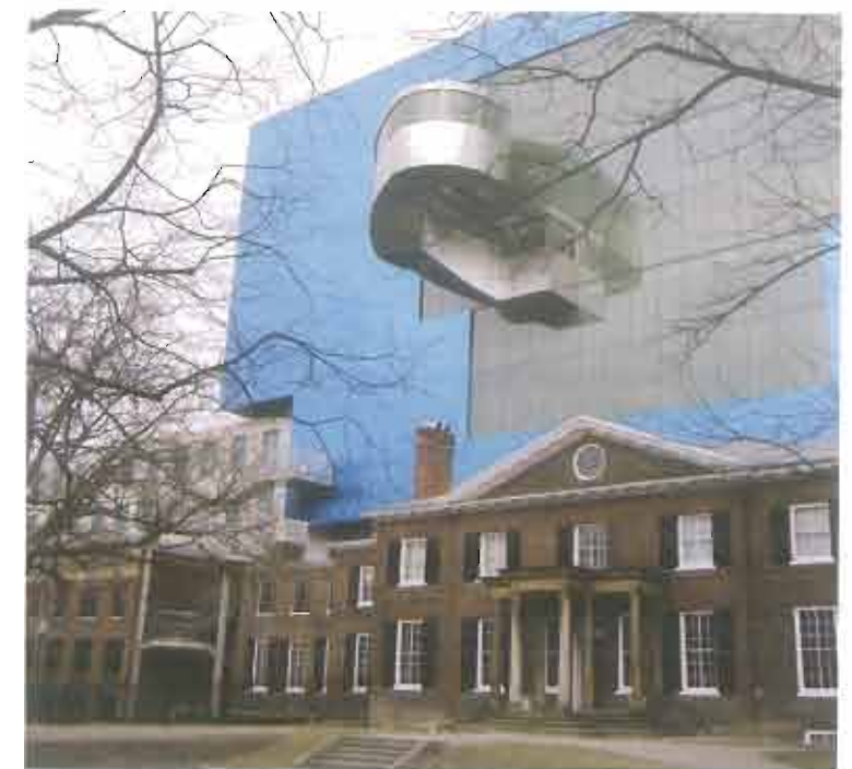
Toronto's Art Gallery of Ontario (AGO) marks the first Canadian building by native son, Frank Gehry. Among its many design features is the striking use of blue titanium and other metals. Use of dissimilar materials can have an impact if corrosion is not taken under consideration.
