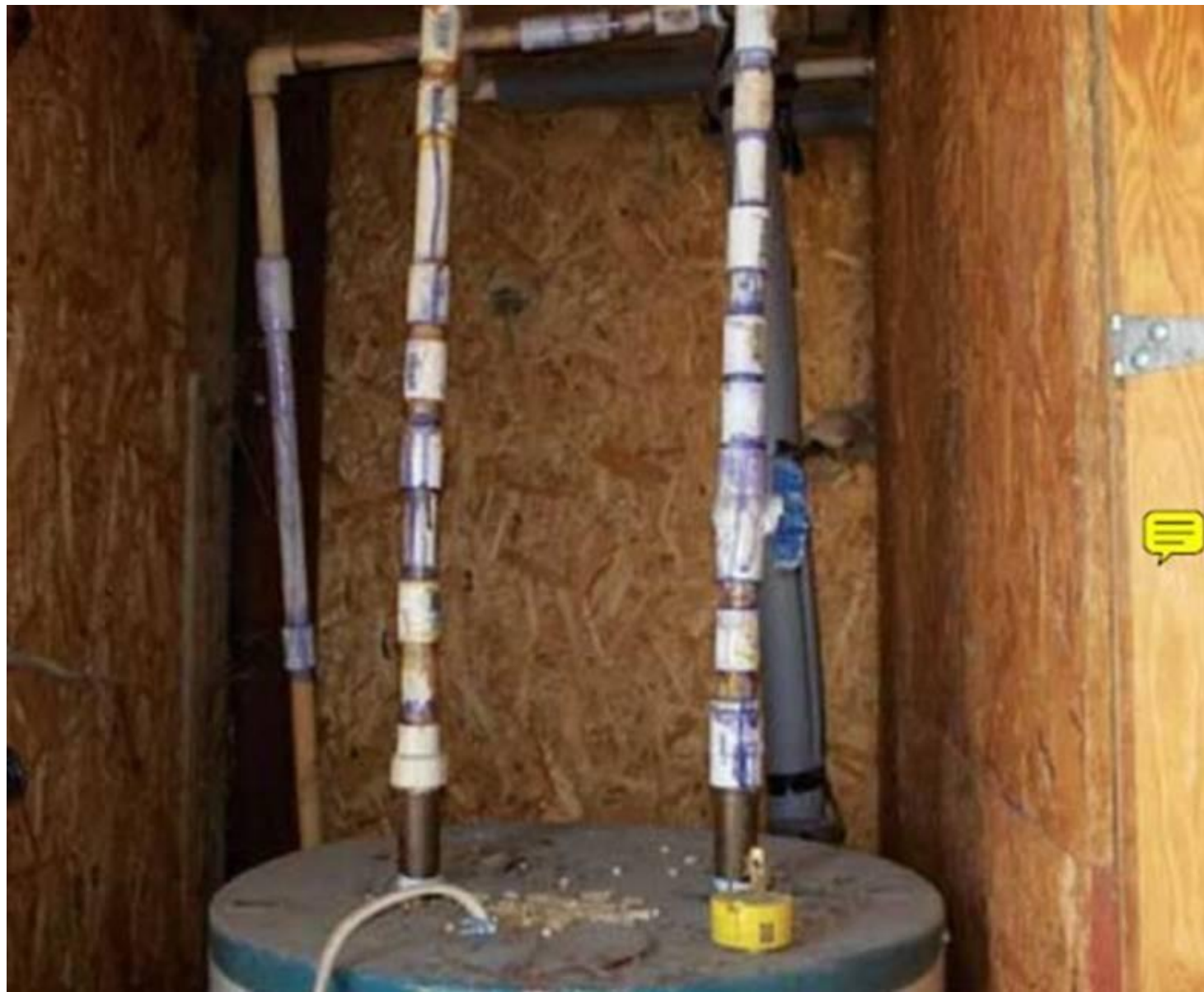
"Look- I had 18" of pipe and this bag of couplers."
