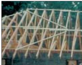
Above: Illustrates use of adequate bracing PHOTO B2-7
