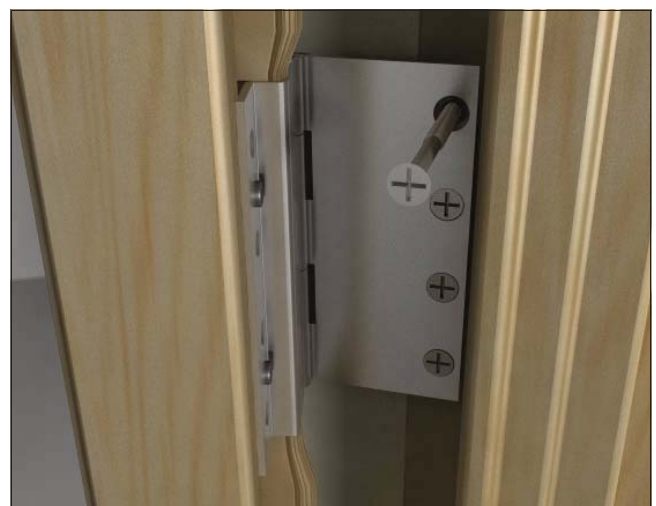
Figure 18 Install screw through butt hinges on UCART.
