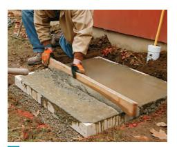
Screed the slab. Flatten the concrete using a straight 2x4 that's about 1 ft. longer than the form width. Move the board forward with a back-and-forth sawing motion while keeping it on the form.
