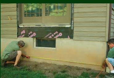
Mark the wall. For accuracy, use a 6, 8, 10 triangle. Mark the wall at 8 ft. from the string.
