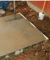
8 Tamp the surface with a rake. Gently tamp the entire surface of the slab. The rake pushes down the gravel that's part of the concrete mix, and brings up a mixture of cement and sand that's easier to smooth.
