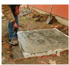
**6** Tap the sides of the form. Lightly hammer the form all around the slab until you see bubbles rising from the concrete. This step makes for a smoother slab edge that won't collect water, which can freeze and spall the concrete.
