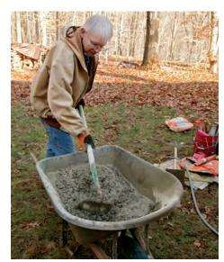
**4** Mix the concrete. Dump two 80-lb. bags of mix in a wheelbarrow for each batch. Add 3 qt. of water per bag, and mix thoroughly with a hoe. Add small amounts of additional water if necessary to bring the concrete to a consistency that's about the same as thick cake batter.
