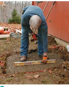
**Grade the gravel.** Fill the excavation  $\checkmark$  with 4 in. of gravel. Rake it flat, and use a level to make sure it's pitched about  $\frac{1}{4}$  in. per ft. so that the slab, which will parallel the base, drains water.
