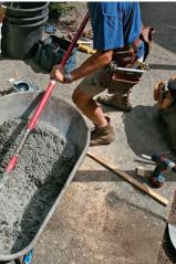
Stand in front to mix. Pull the concrete to the front, and water will flow in behind it. Because I'm standing at the front of the wheelbarrow, I can now work the concrete without having the wheelbarrow move as I push back and forth. Let the water flow in after each push-and-pull stroke. Keep mixing until most of the water is absorbed.
