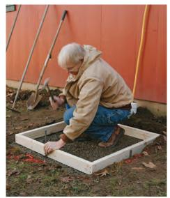
**3** Make and set the form. Most 4-in. slabs are actually the 3<sup>1</sup>/2-in. depth of standard 2x4s. Nail the corners together, and place the form on the graded gravel, making sure it doesn't rock. Drive 12-in. lengths of rebar to just below the top of the form to keep it from moving.
