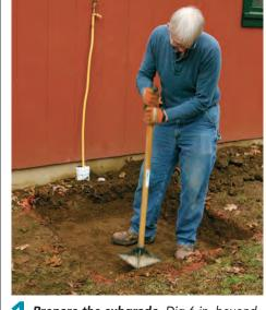
**1** Prepare the subgrade. Dig 6 in. beyond where you want the slab edges and 8 in. deeper than where you want the top of the slab. Make sure the subgrade pitches away from the building, and tamp down loose soil.
