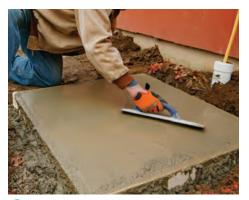
Smooth the rake marks with a mag **7 float.** Keep the leading edge of the float up. When the surface water dissipates, float the slab again. This is the final finish for exterior slabs. For a smooth interior slab, work it again with a steel float when the surface begins to lose its wet sheen.
