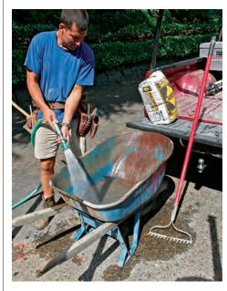
**2** Add the concrete. Place the unopened bag in the water. Then use a utility knife to open the bag with a single cut along the end. Grab the bottom of the bag and tip it up so that the concrete slides out rather than pours out. This technique minimizes dust.
