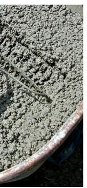
wet and I've scraped the rake along the bottom and sides to remove any dry pockets. The mix passes my personal slump test when it's all wet but still firm
