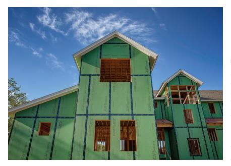
The ZIP System® portfolio of wall and roof solutions offers structural panels in a range of thicknesses, lengths and even R-values, thanks to the line of ZIP System® R-sheathing panels with integrated exterior insulation providing R-3 to R-12 thermal resistance.
