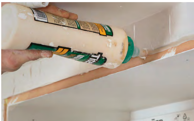
Bond with glue. Apply a bead of glue (we use Titebond III) on the MDF, close to the outside edge, to bond the paper tape to the return.
