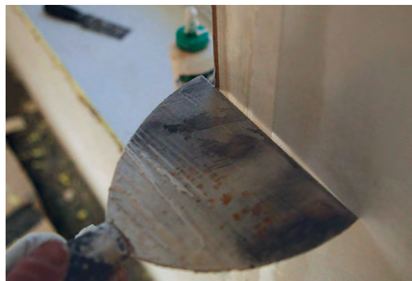
Set it back. Embed the paper tape in the glue and compound, centering the edge of the tape on the MDF to prevent it from showing through after the finish coats are applied.
