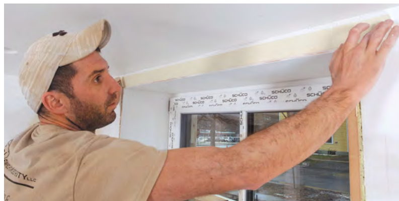
Set it back. Embed the paper tape in the glue and compound, centering the edge of the tape on the MDF to prevent it from showing through after the finish coats are applied.
