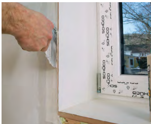
Bond with glue. Apply a bead of glue (we use Titebond III) on the MDF, close to the outside edge, to bond the paper tape to the return.
