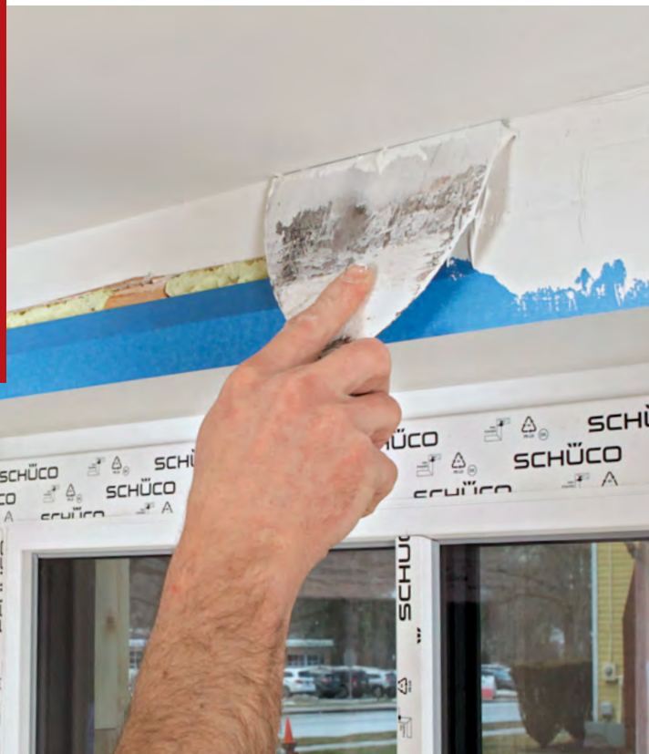
Compound first. Starting at the top, apply all-purpose joint compound over the foam and onto the drywall, being careful not to get compound on the MDF. In tight spaces, painter's tape keeps the MDF clean.
