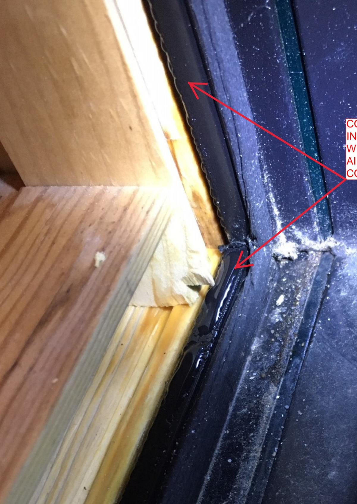
CONDENSATION ON INSIDE OF WEATHERSTRIP. WARM AIR CONDENSING ON COLD FRAME.
