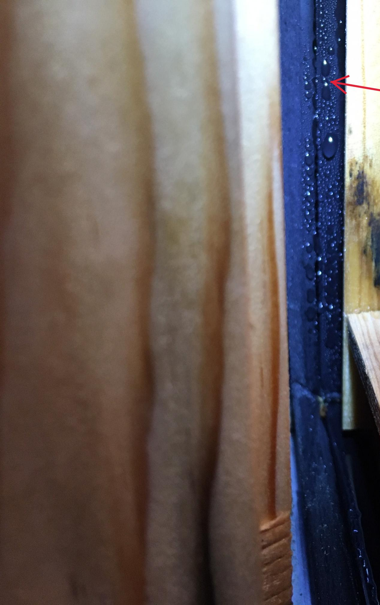
WATER CONDENSING ON INTERIOR SIDE OF WEATHERSTRIPPING. WATER TRAPPED AND STAINS WOOD FRAME.
