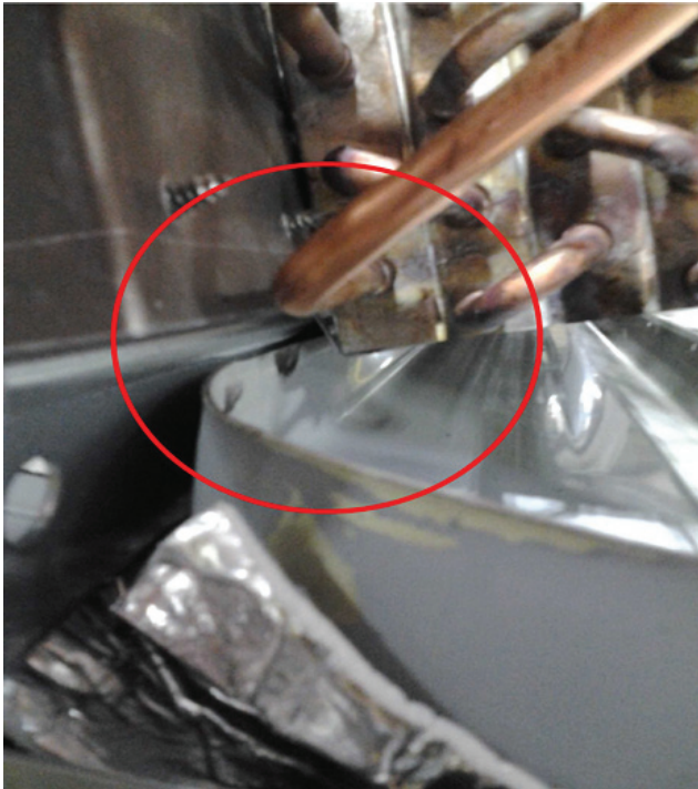
Figure 4. A mis-aligned grommet does not allow for proper drain pan position
