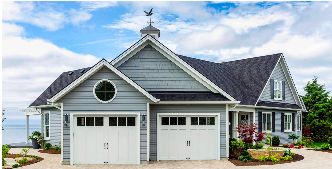
High wind pressure on coastal homes and other inclement-weather areas has resulted in increased wind-resistance requirements for garage doors.
