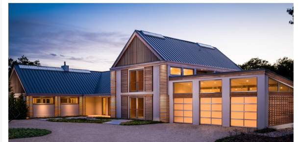
Aluminum frames holding glass panels depart from suburbia, providing a sleek, urban aesthetic.
