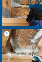
nozzle, so keep steady pressure on the trigger. Spray the cavity perimeter first, then cross back and forth to fill the space. Adjust the speed of your strokes to get the thickness you're looking for.
