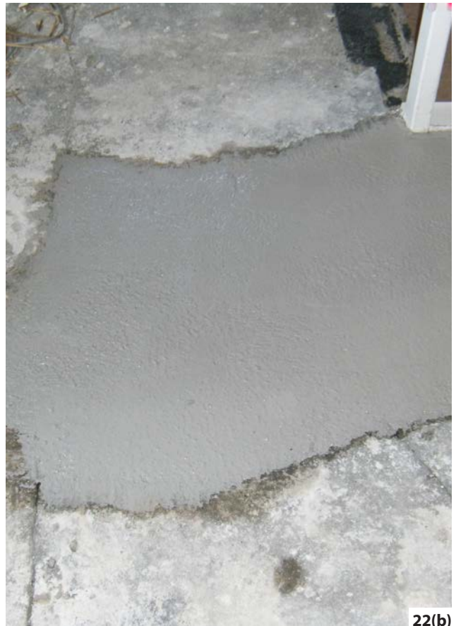
Figure 22: Patch repair: (a) New plaster being spread over a dressing of lime putty. (b) Finished level with the existing surface. Photos: A J Goode Ltd
