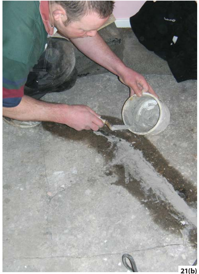
Figure 21: Cracking in gypsum plaster: (a) Raked out for repair. (b) Filled with a matching new mix. Photos: Douglas D Kent (a) and A J Goode Ltd (b)
