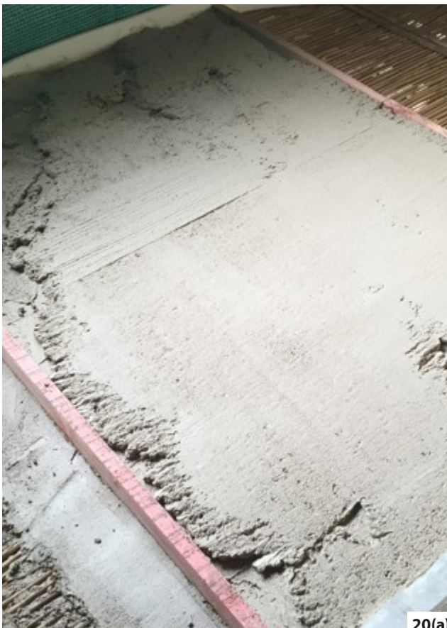
Figure 20: New gypsum plaster being laid between temporary timber battens (a) before the adjacent sections are infilled (b).
