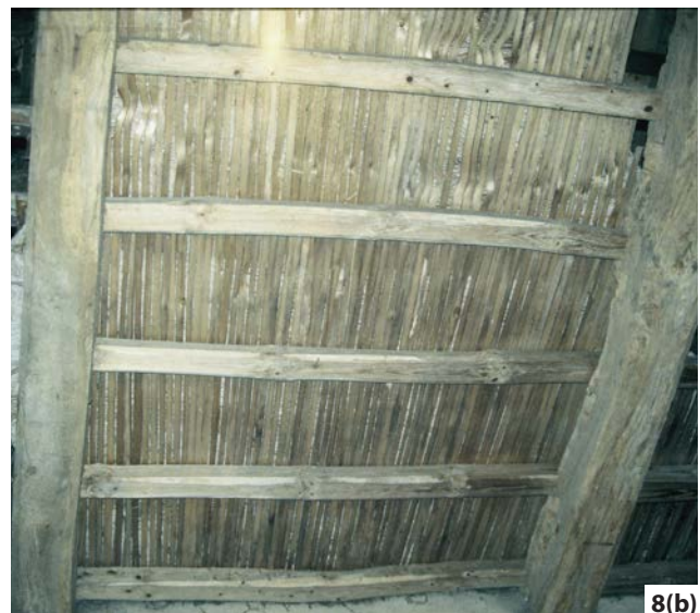
Figure 8: Organic bedding material: (a) Reed, as seen in a sample box cutaway. (b) Laths.
