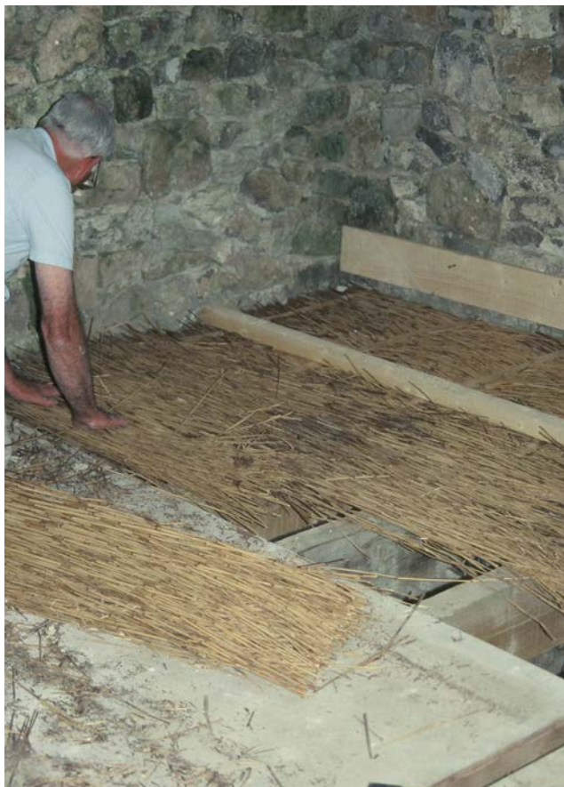
Figure 17: New reed bedding being laid.
