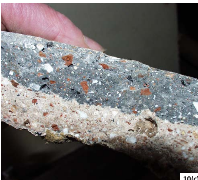
Figure 10: A historic solid gypsum plaster floor at Scraftoft, Leicestershire laid to imitate tiles: (a) General view. (b) Alternating black and white 'tiles'. (c) The two layers forming a black tile. Photos: A J Goode Ltd
