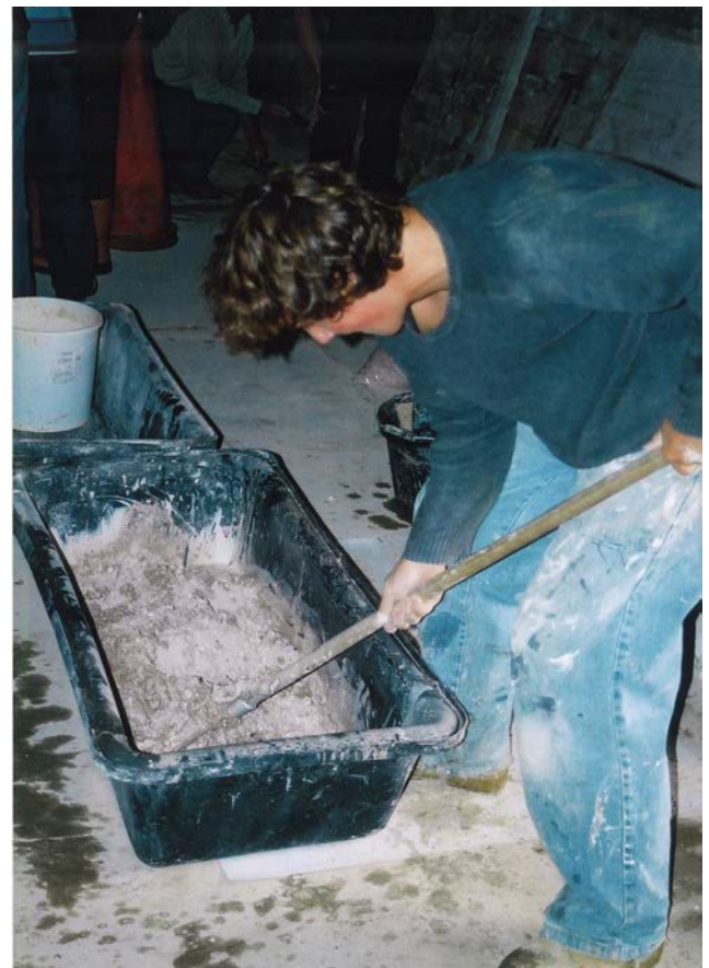
Figure 19: Mixing gypsum plaster in a plasterer's bath. Photo: Douglas D Kent
