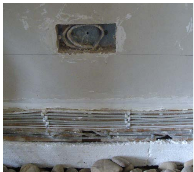
Figure 9: A stone base for a new gypsum plaster ground floor.
