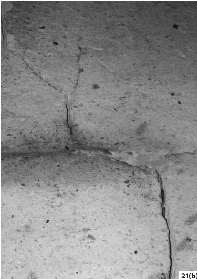
Figure 21: Cracking in gypsum plaster: (a) Raked out for repair. (b) Filled with a matching new mix. Photos: Douglas D Kent (a) and A J Goode Ltd (b)
