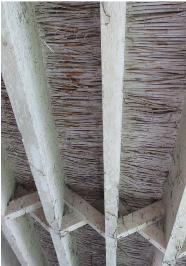
Figure 2: The presence of organic bedding material, such as reed, can indicate the existence of a gypsum plaster floor.
