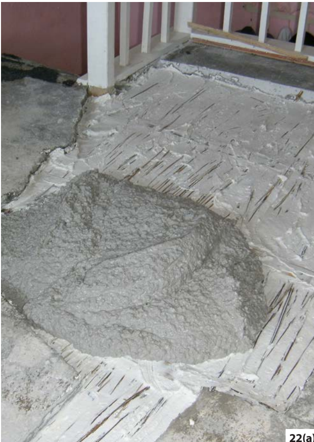
Figure 22: Patch repair: (a) New plaster being spread over a dressing of lime putty. (b) Finished level with the existing surface. Photos: A J Goode Ltd
