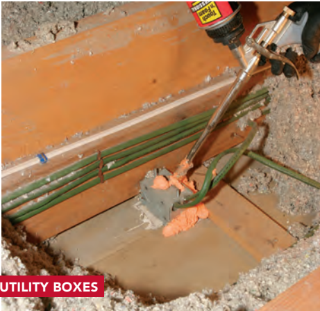
PENETRATIONS IN WALL PLATES
