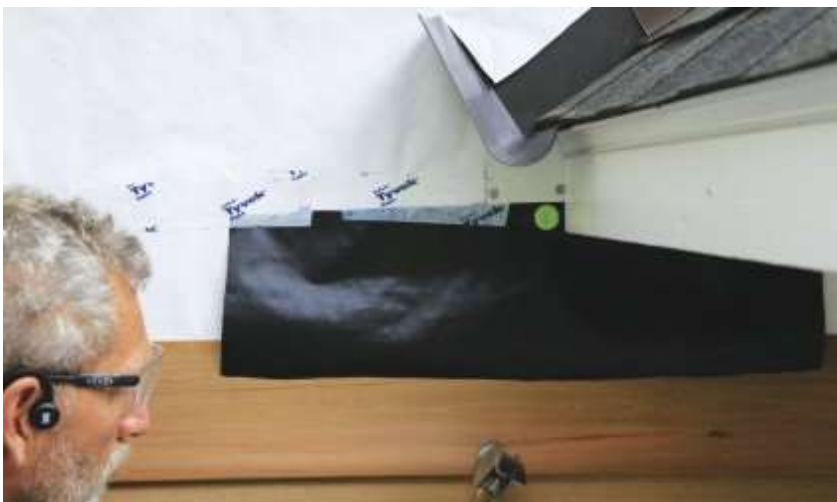
Anchor the top and sides of this last piece of WRB, sealing it to the main WRB. Leave gaps in the tape at the bottom to allow any water to escape.
