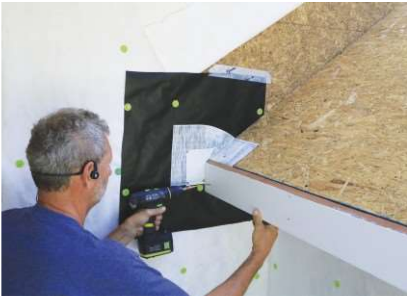
The finished fascia goes in next.
