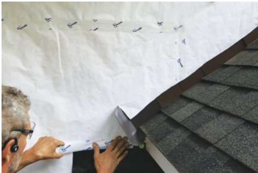
Anchor the top and sides of this last piece of WRB, sealing it to the main WRB. Leave gaps in the tape at the bottom to allow any water to escape.
