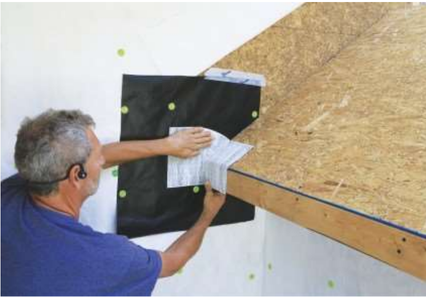
Flexible flashing tape bridges the intersecting surfaces.
