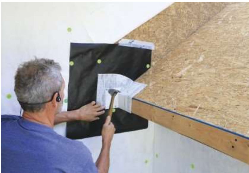
Metal flashing protects the tape.
