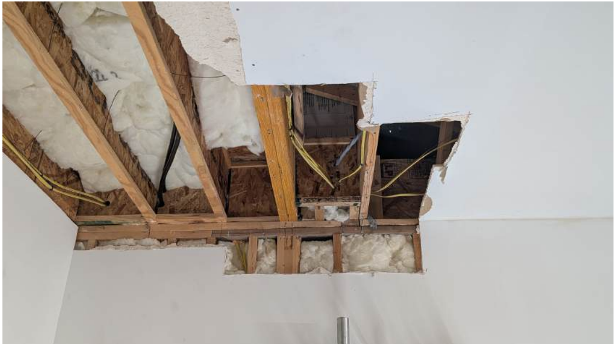
-Living space common walls, living space above. Open space to front porch awning connected to garage attic on the right.
